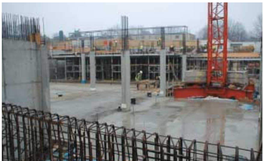
Building progress on the Cancer Genomics Centre
