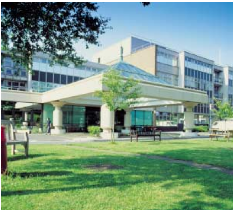
Below: The new Royal Marsden building at Sutton
