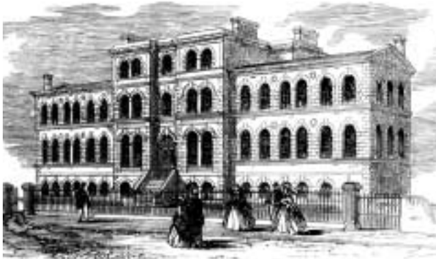
The new Cancer Hospital at Brompton, 1862
